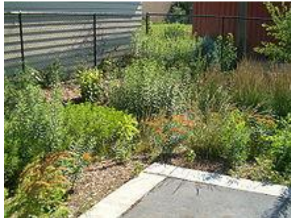
business parking lot with rain garden to absorb rainwater runoff
